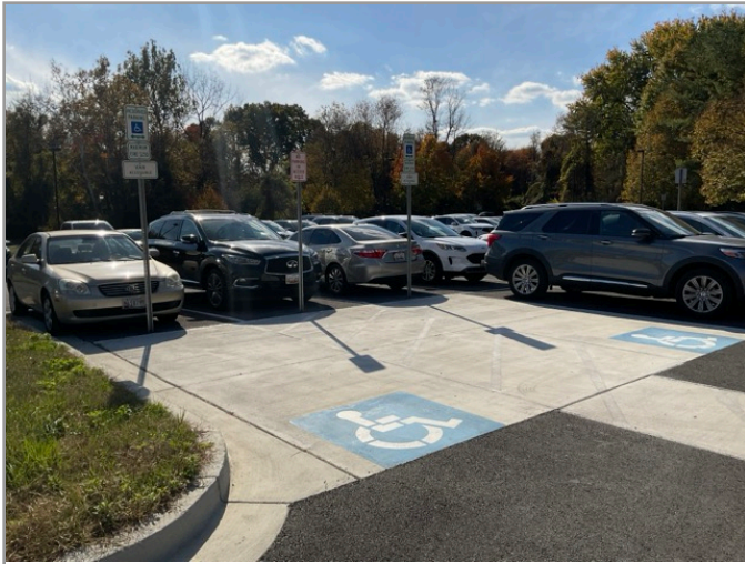
OVERVIEW OF ACCESSIBLE PARKING AREA
