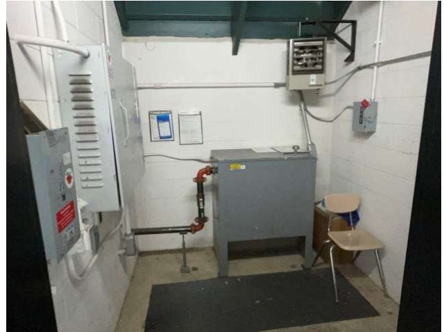
26 - ELEVATOR MACHINE ROOM
