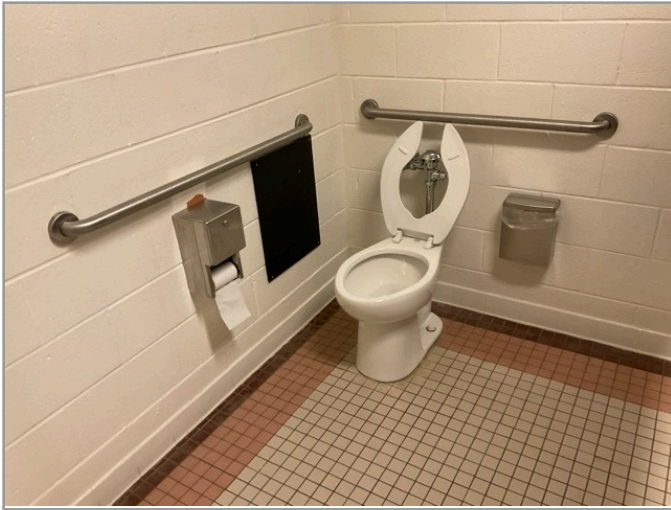
TOILET STALL OVERVIEW
